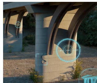
Inspection of infrastructure
