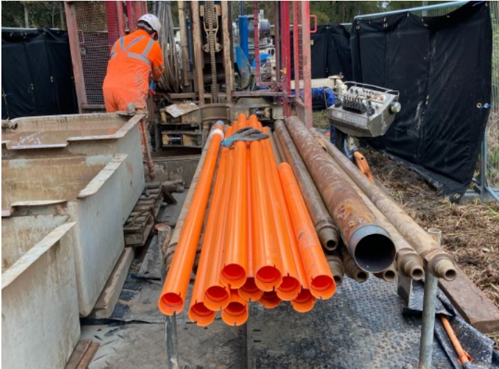
Inclinometer casing awaiting installation
