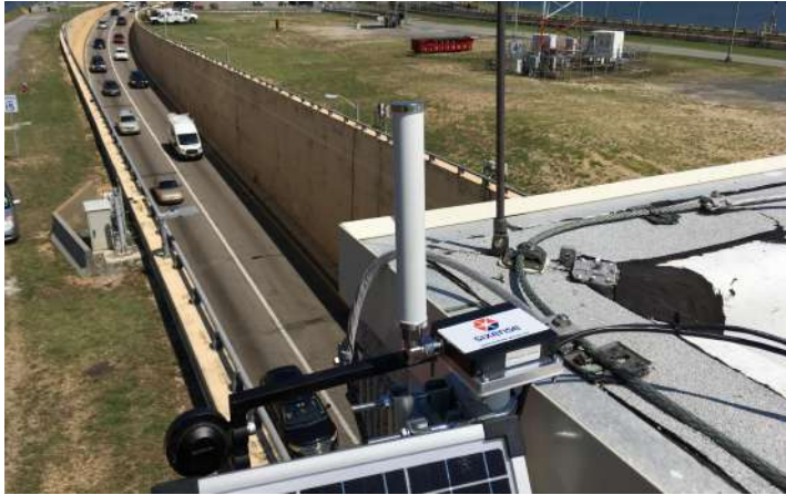
4DBloc - GNSS sensor installed on site
